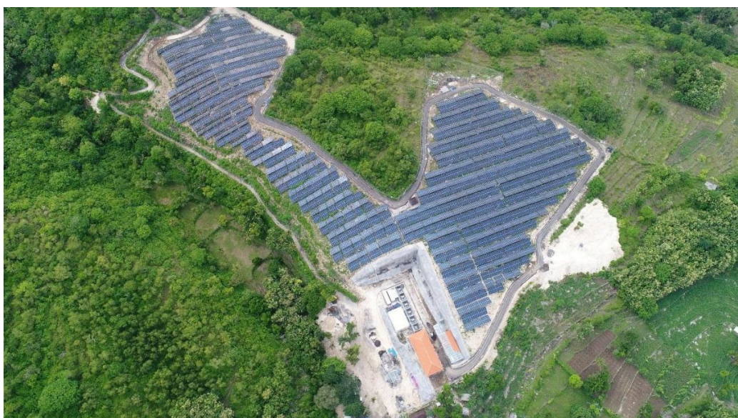
Nusa Penida Solar Power Plant Facility
