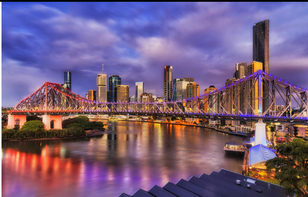
The Story Bridge in Brisbane, QLD - Australia.
