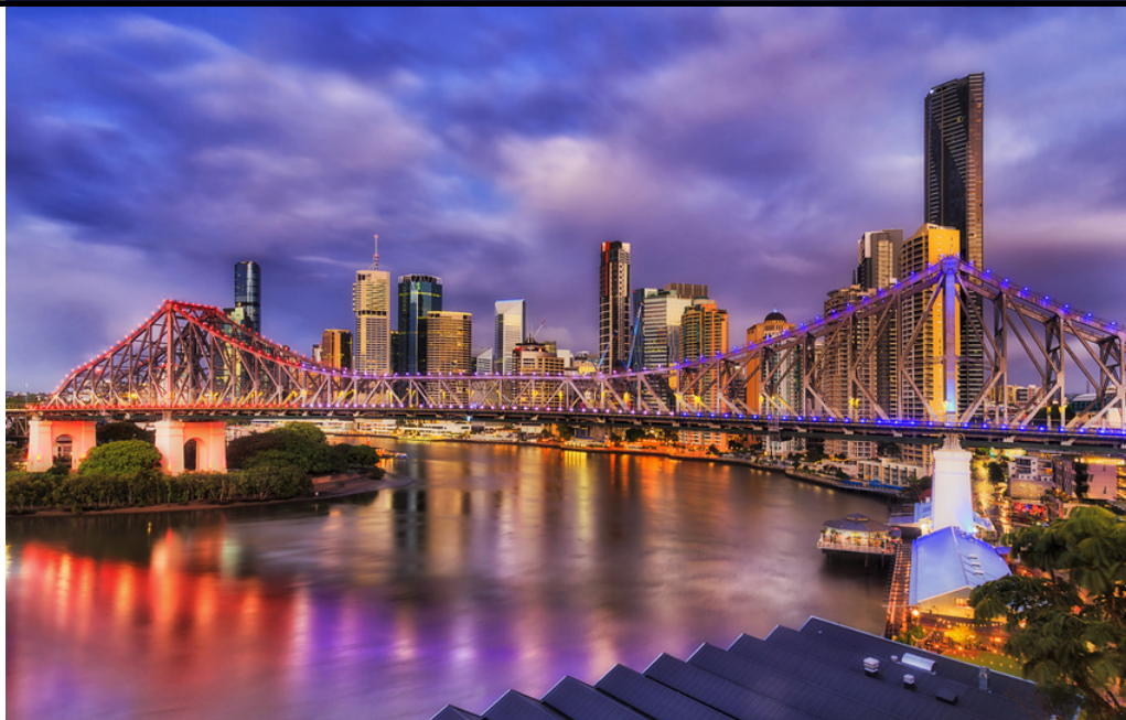
The Story Bridge in Brisbane, QLD - Australia.
