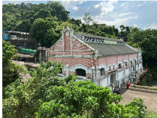
Panoramic view of Xiaocukeng Power Plant
