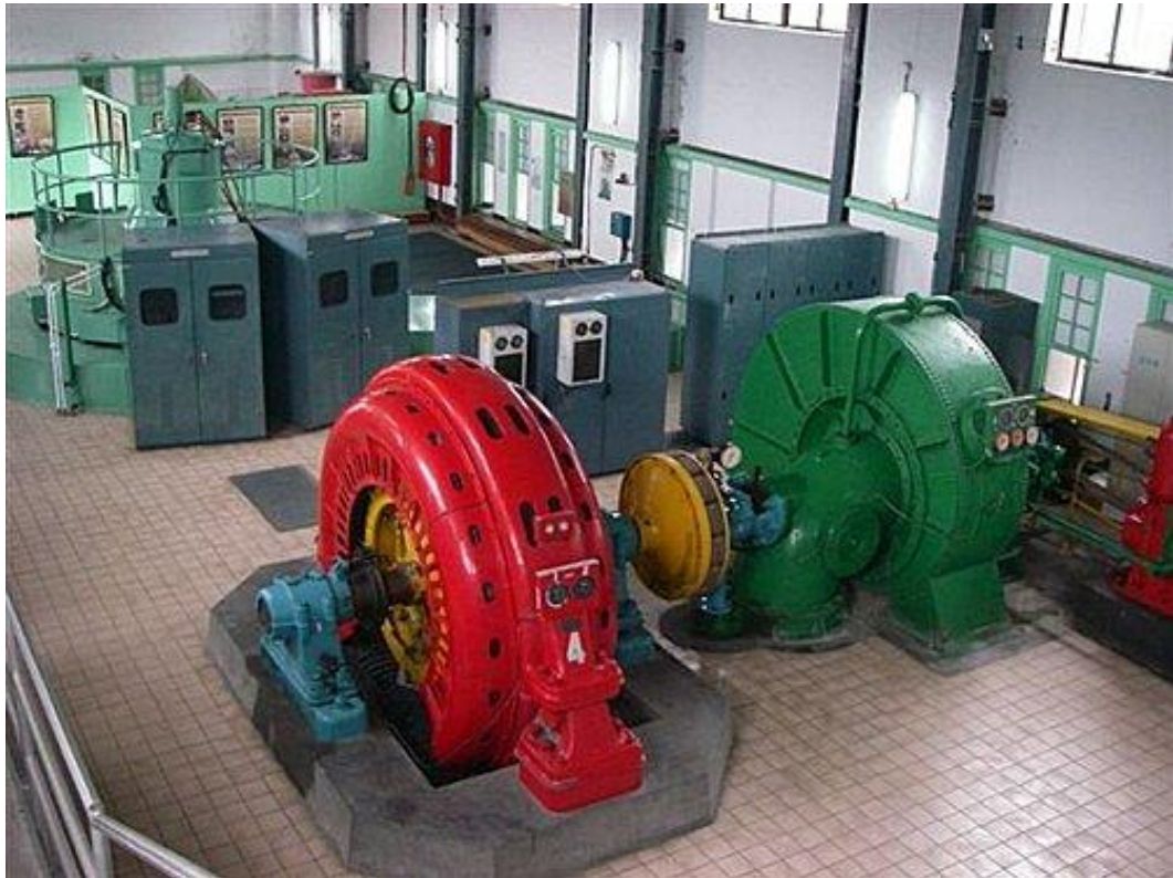
View of the Generators and water turbine
